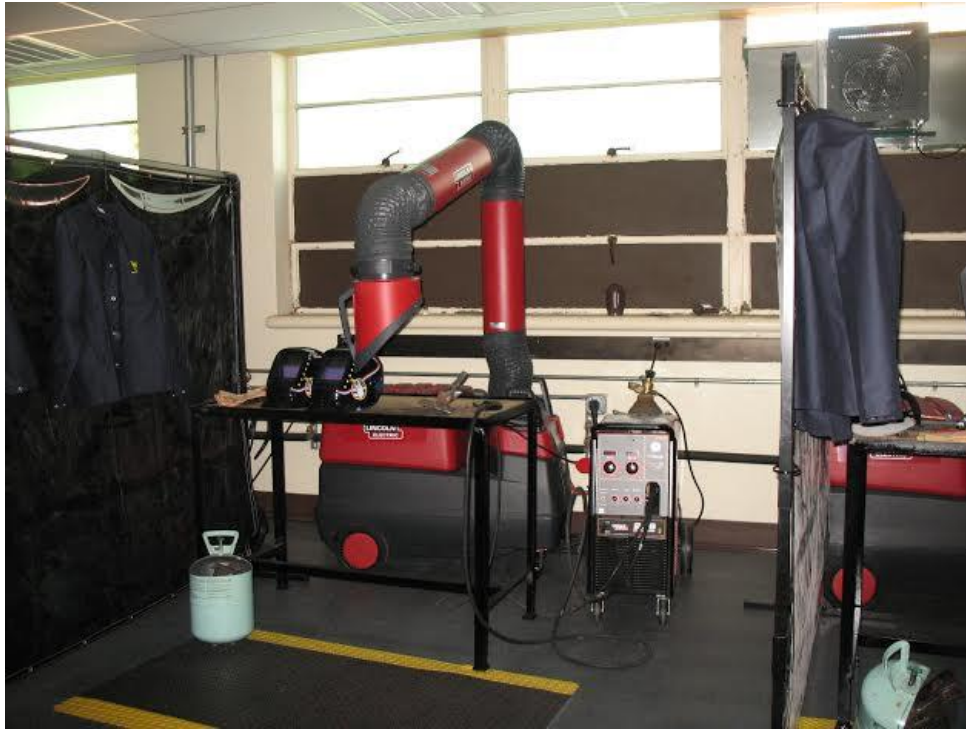
Figure 1.7 Mechanical Engineering Fusion Welding Laboratory
